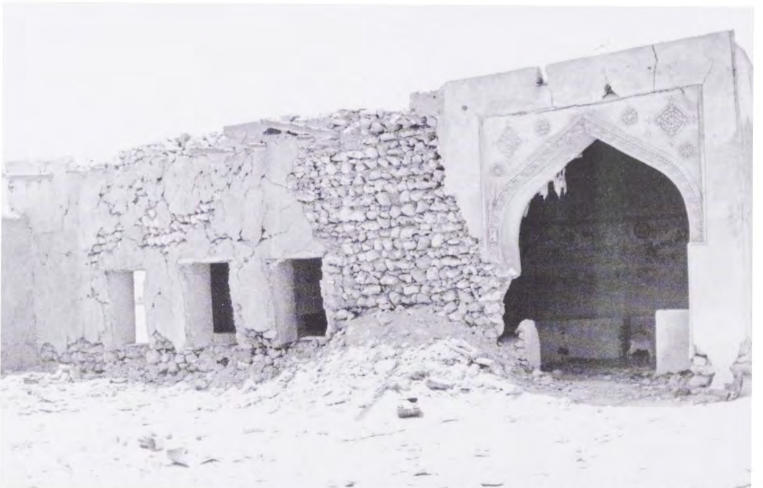
(Fig. 6) : Eastern gate before restoration.
